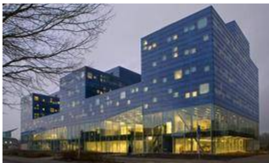
Figure 1.1: The Bernoulliborg building.
